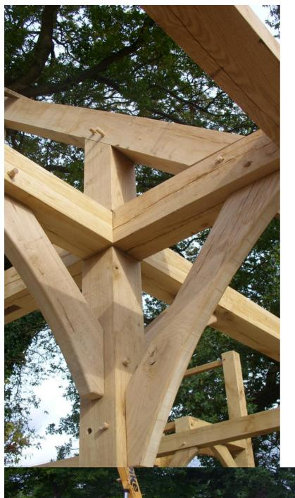
Fast growing oak is structurally stronger than slow growing oak. The vessels (the rings we count to determine the age) are further apart resulting in the fibres being longer and more dense, and the denser the fibres the stronger the beam will be. The fibres give the trunk its strength. All our frames are planed and sanded with all sharp edges removed. The joints are traditional mortice and tenon, held in place by seasoned oak
